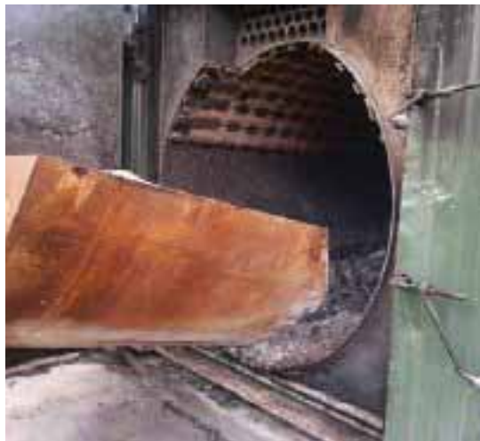
The Skelhoje boiler, installed on Jimmy Foran's farm, being cleaned out by a specially-designed bucket.
